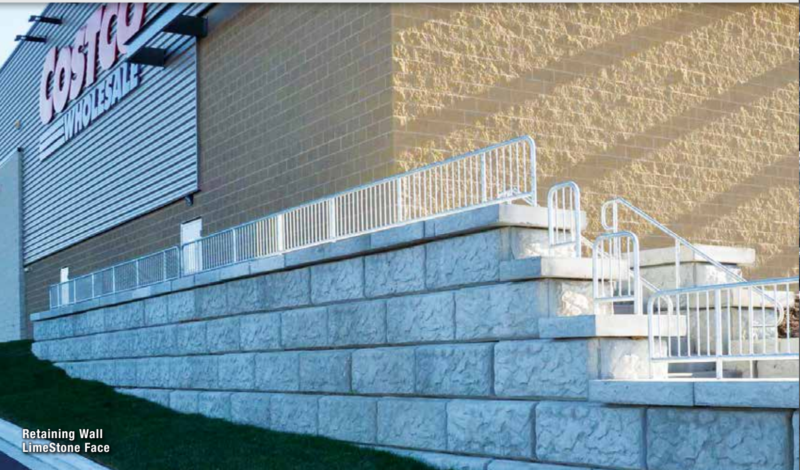
Retaining Wall CobbleStone Face / Stained
